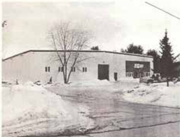
VTrans Collections Storage Facility, East Montpelier
