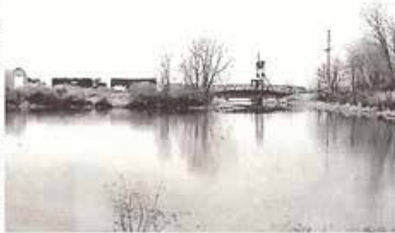
North End of Barge Canal
